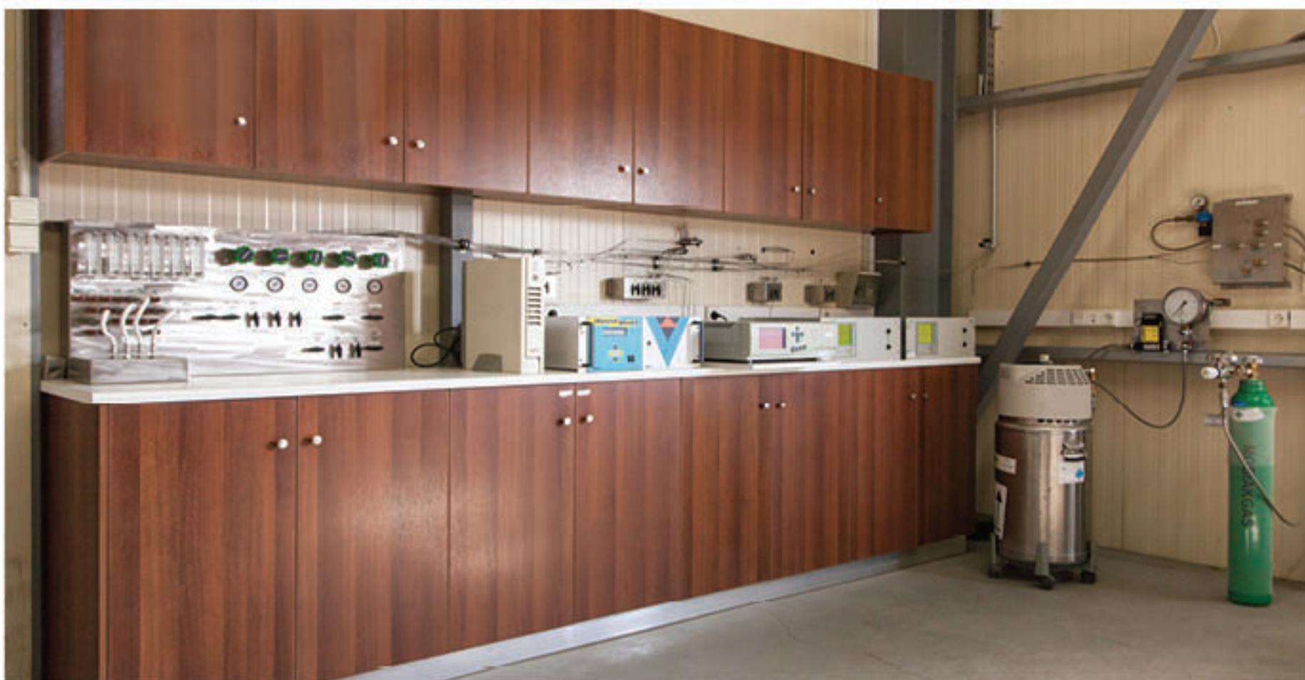
Chemical Laboratory Equipped with Quality Control, Gas Analysis Fire Extinguishing Agent Analysis Instruments
